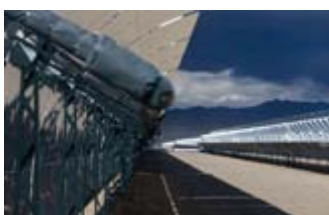
The Nevada Solar One CSP power plant near Las Vegas, Nevada. The 400-acre, 64 MW CSP plant produces enough energy to power about 14,000 homes (Photo: Reuters)
